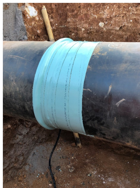
Figure 2: Sensors covered with protective coating
